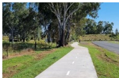
Image 25. Shared path with landscape buffer to road.
