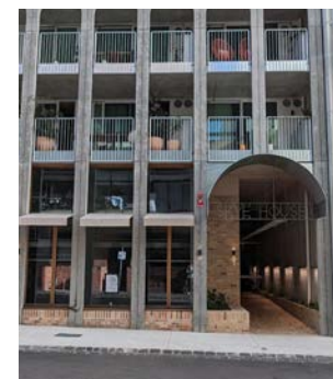
Image 43. Visibility for passive surveillance of the street.
