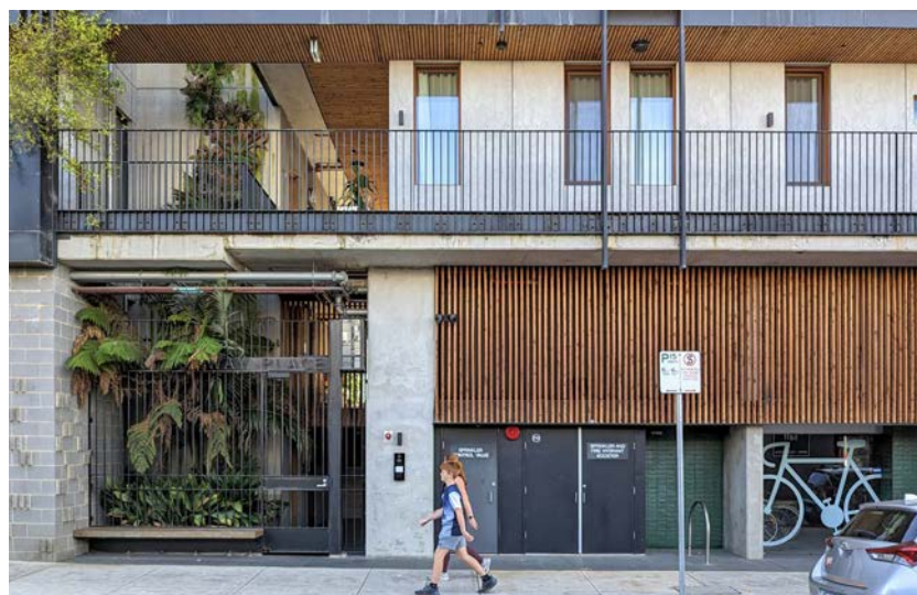
Image 45. Landscaped entrances with passive surveillance above.
