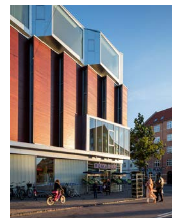
Image 46. Active ground floor corner of building.
