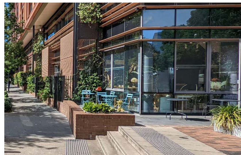
Image 41. Active frontage and glazing, surrounded by landscape.
