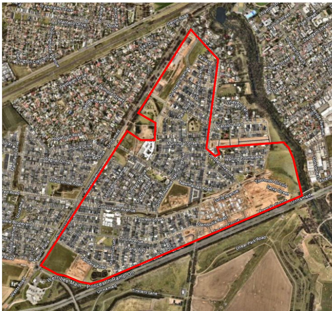
Figure 2: Aerial photo of Riverwalk Estate (January 2026)
